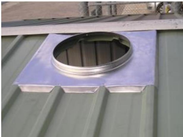
Shape flashing base to roof profile and secure base, preferably under ridge capping
