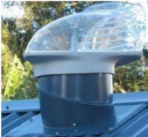
Secure head of unit by lining up pre drilled brackets and fix with screws provided
